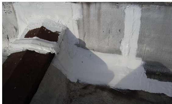
Coping Tile Repair (After)
