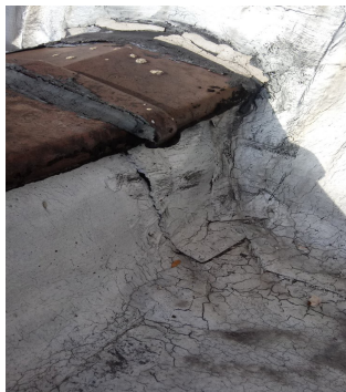
Coping Tile Repair (Before)
